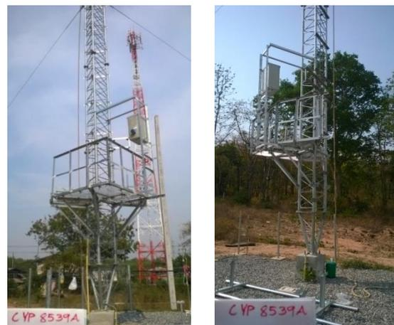
Figure 3. Platform of mobile device transmitter
